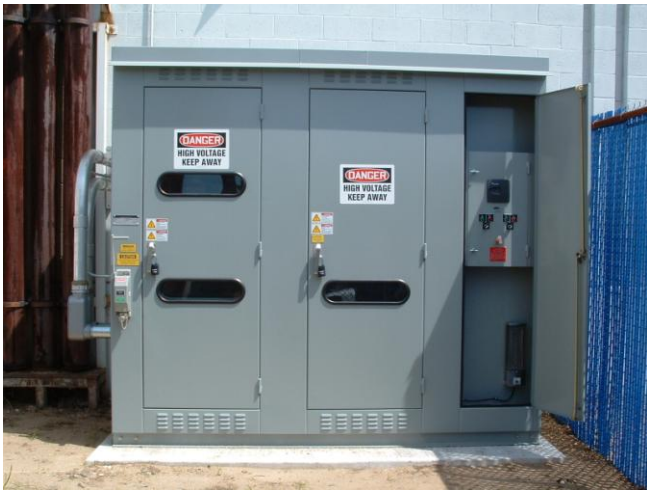
This is an example of one of our pad mounted 13.8 kV automatic power factor correction units.
