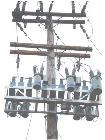
This is an example of one of our pad mounted 13.8 kV automatic power factor correction units.
